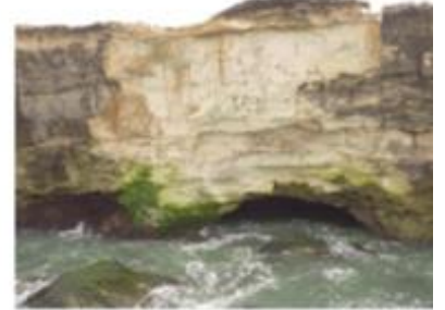
CAVE & CLIFF COLLAPSES
